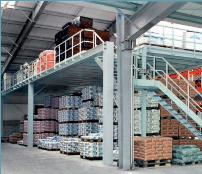
Storage platform in the building materials trade. Storage area up to the warehouse roof. Placement of the stairs outside, with pedestal and railings in steel/steel construction.
