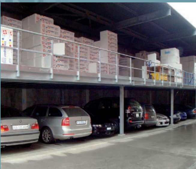
Hot dip galvanized steel construction platform for outdoor use. Use of the bottom floor as parking spaces.
