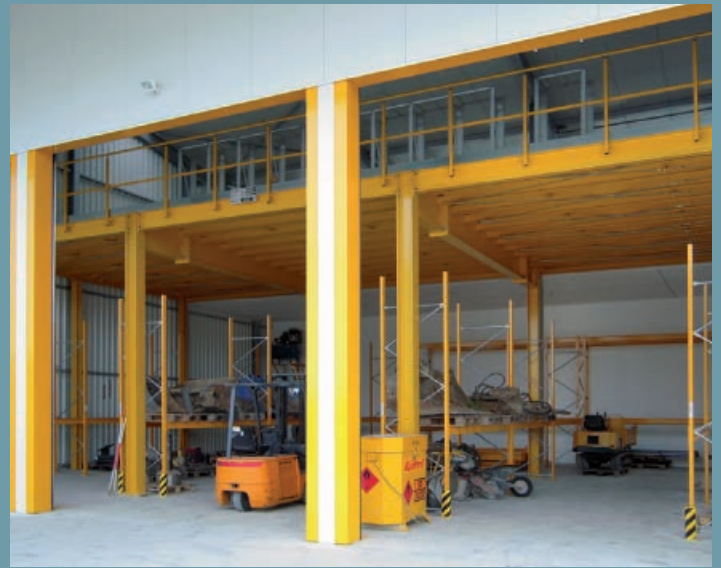
Tailored to the existing warehouse dimensions. Storage platform with racks beneath and on top of the platform.
