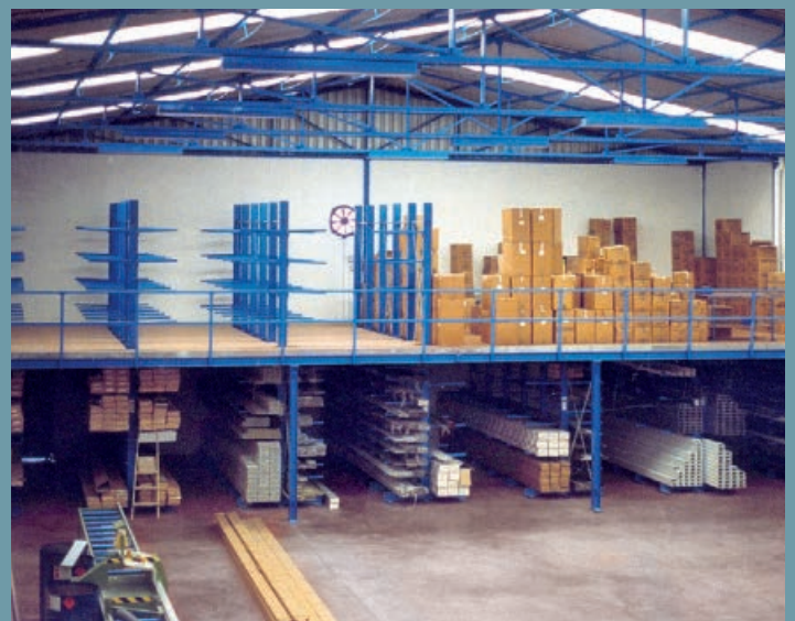
Storage platform with cantilever racks as mezzanine floor. Top packaged goods storage and partial racking.
