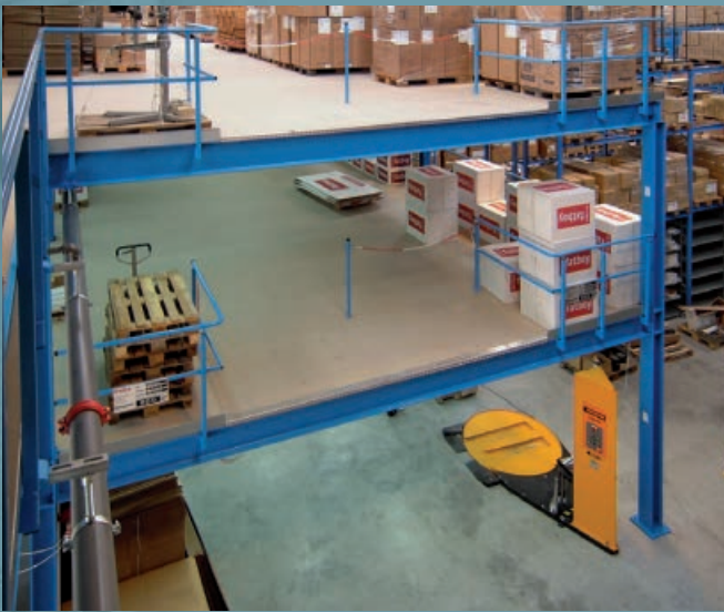
In a multi-storey storage platform. Wholesale distributor. Storage of more than 5000 articles, preparation and order picking on a minimal footprint.
