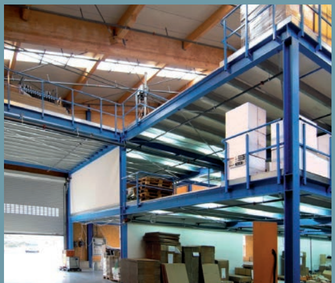
Storage and picking on 3 levels. Maximum possible use of the existing storage area including a tier above the gate.
