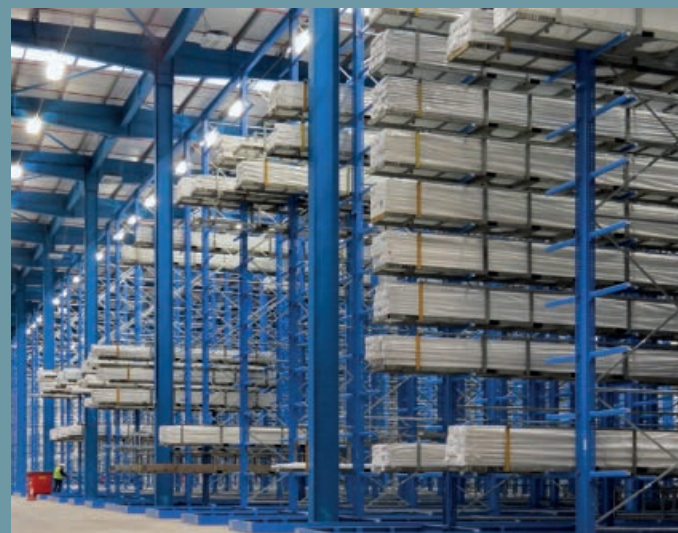
Cantilever racking warehouse 13,500 mm tall with 13 arm levels for aluminium and plastic profiles, which are stored in stillages.
