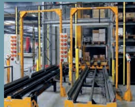
Before the handover to the storage and retrieval machine the materials are measured by means of an electronic contour check, and stock control is documented
