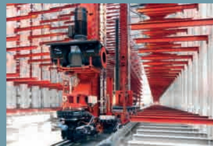
Rack riser truck during a test drive in the empty warehouse
